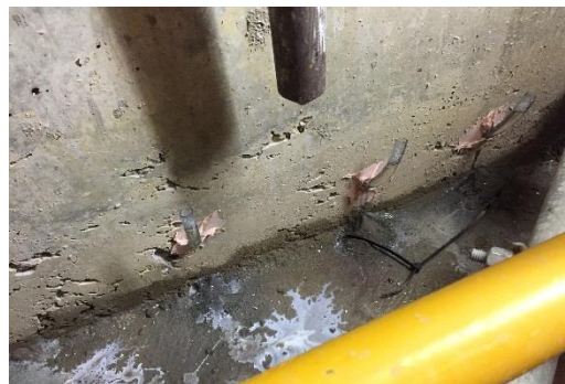
Installing ports
