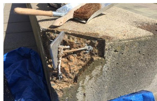
Breakout and steel install
