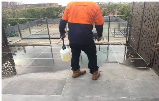
Applying Silane Spray
