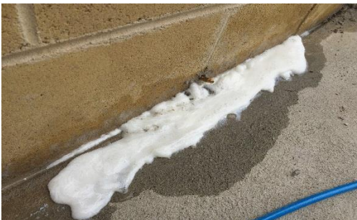
PU reacting with water
