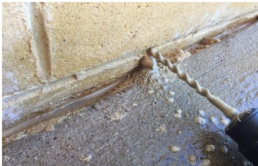
Drilling holes for injection
